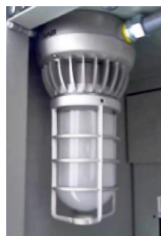
Figure 3. LED jelly jar with heat-dissipating design.
