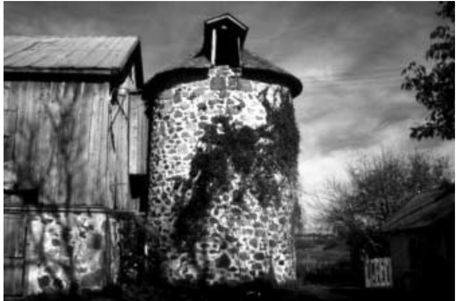
Stone silo built circa 1900. Manitowac County.
