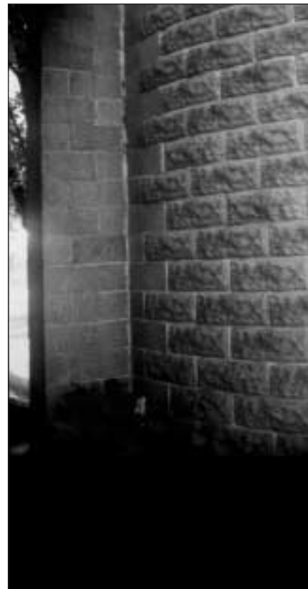
Rock face and plain concrete blocks in a Jefferson County silo.
