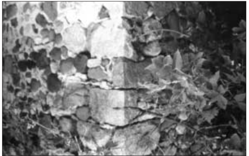
Square stone silo. Waukesha County.
