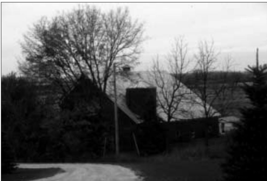
Wood stave silo. La Crosse County.
