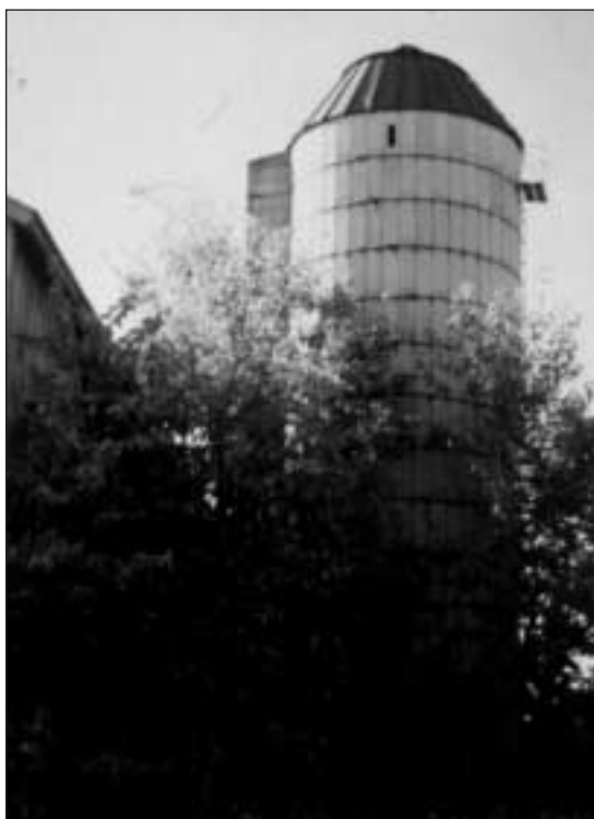
Concrete stave silo, built before 1919 in Walworth County.
