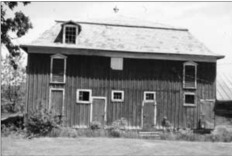
Barn of A. A. Arnold, Trempealeau County. Interior silo is filled through the dormer on the left.
