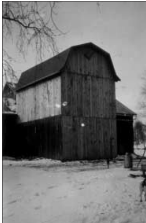
Silo built by John Hays in 1882 in Dodge County. Stone with wood jacket. College of Agriculture Archives.
