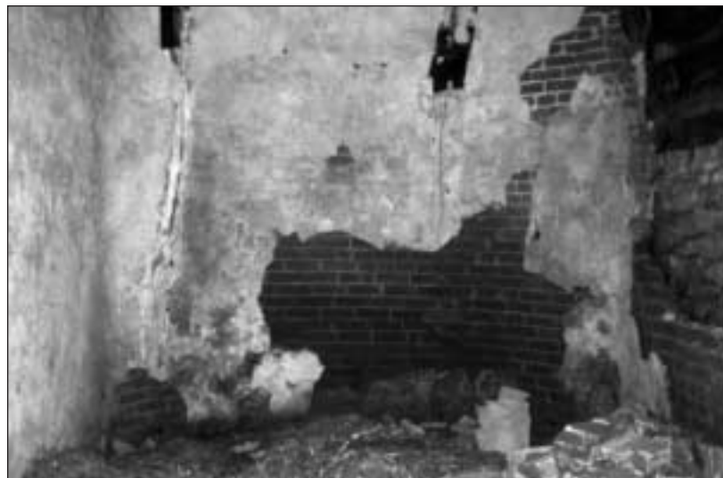
Arnold's interior silo, constructed in 1887 of brick with a cement lining.
