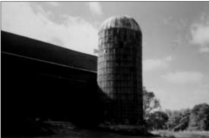
Tile stave silo. Jefferson County.
