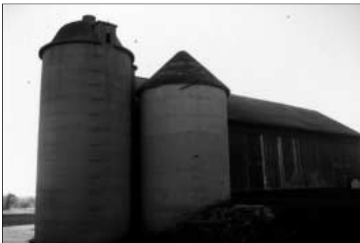
Two monolithic concrete silos. Fond du Lac County.
