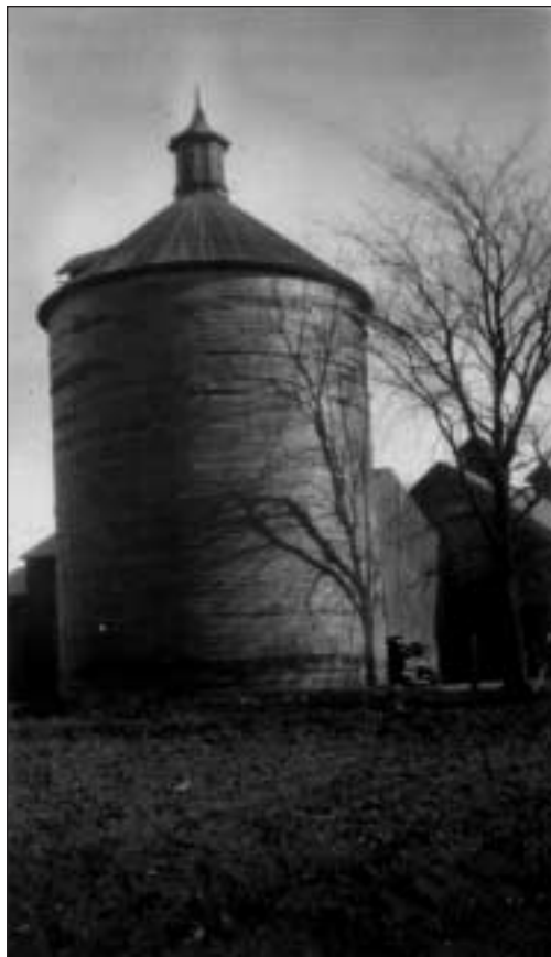
King silo built in 1899 near Racine. The silo is 36 feet tall with a diameter of 24 feet.
